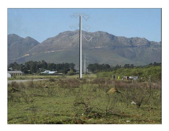
**Photograph 2.1:** Monopole structure which can be used in areas where there are space constraints
